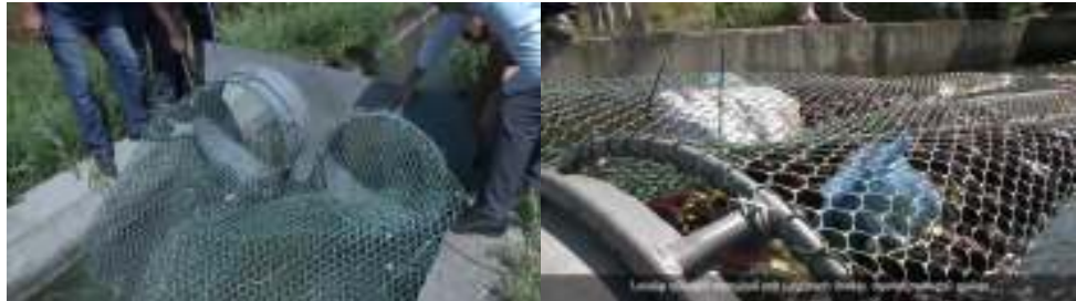
“Trap for Trash” in irrigation canals
